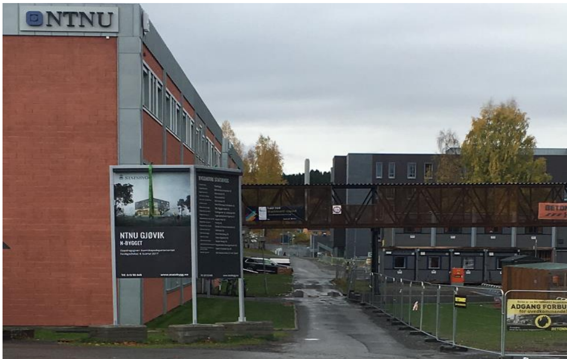
Figure 3: View of Eidsiva Plant from NTNU University (October, 12, 2017).
