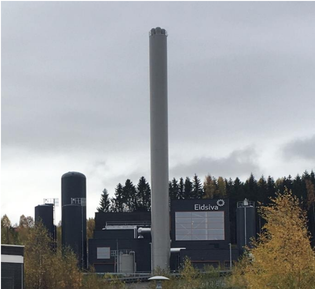
Figure 1: The Eidsiva Plant (October 9, 2017).
